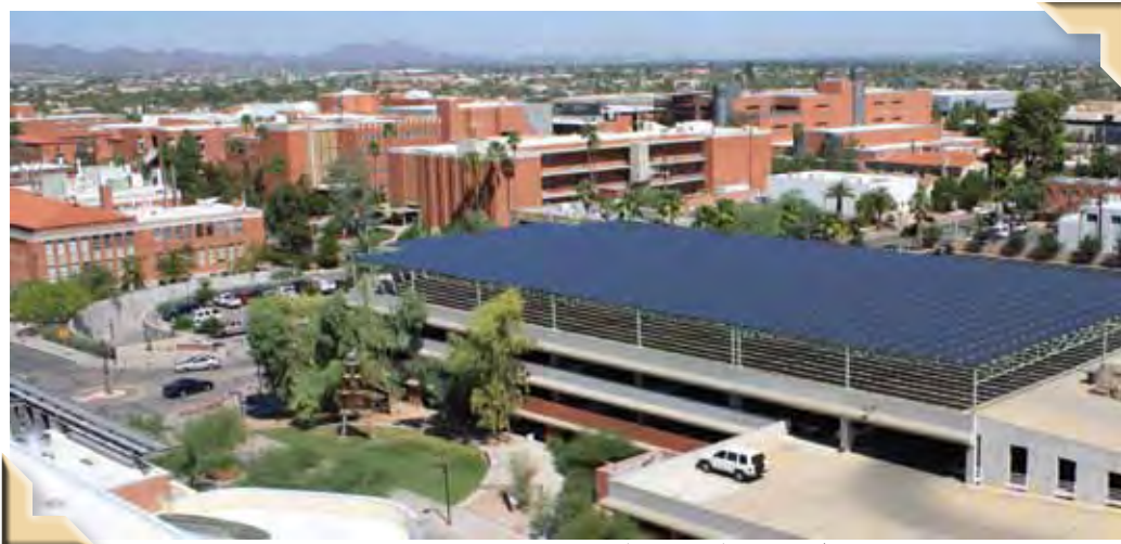
Solar panels atop the Second Street Garage LESLIE JOHNSTON
