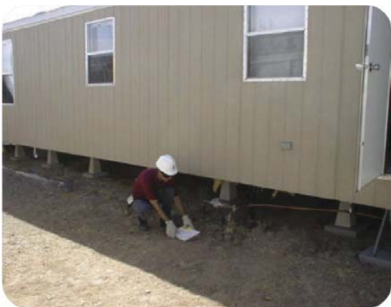
Photo 1: Department employee conducting an installation inspection
